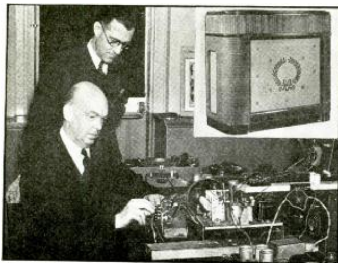
Interior of radio station W2XMN atop the Palisades (N. J.) near the George Washington Bridge; this transmitter employs frequency modulation. Static-less radio programs will soon be transmitted, on 40 mc. (about 7 meters), over a service area of about 100 miles. Control desk is shown in foreground.
